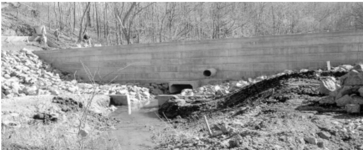
Detention Basin B Dam Under Construction
