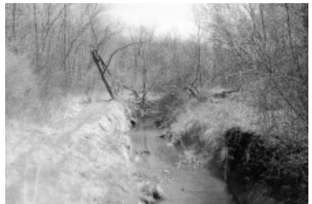
Zimber Ditch Dam Location Before Construction
