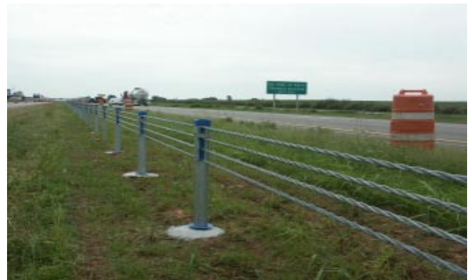
Safety Cables Along Interstate
